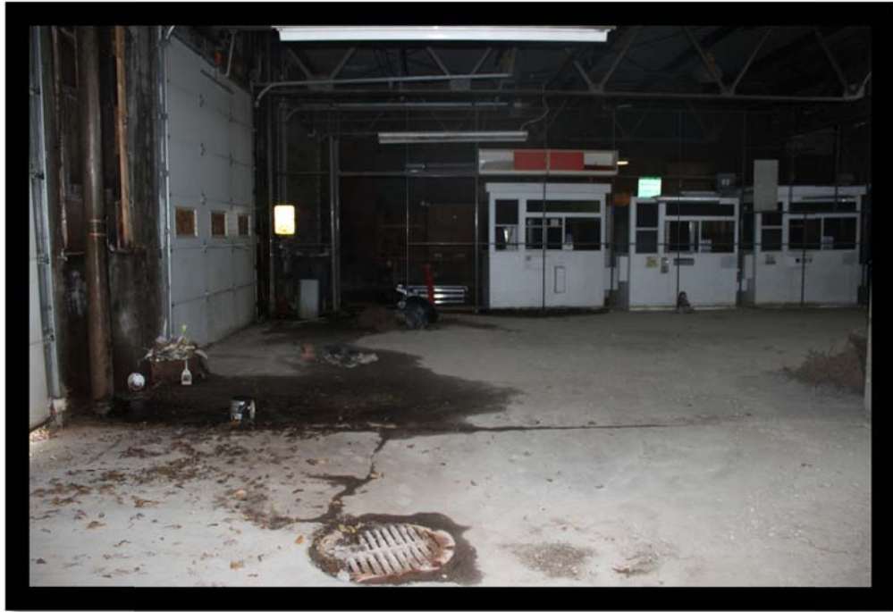
Looking south at the former "lawn mower repair" area of the West Garage
