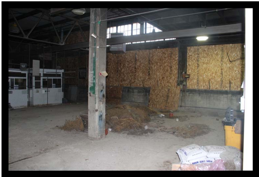
Looking west at the former "radio repair" area of the West Garage
