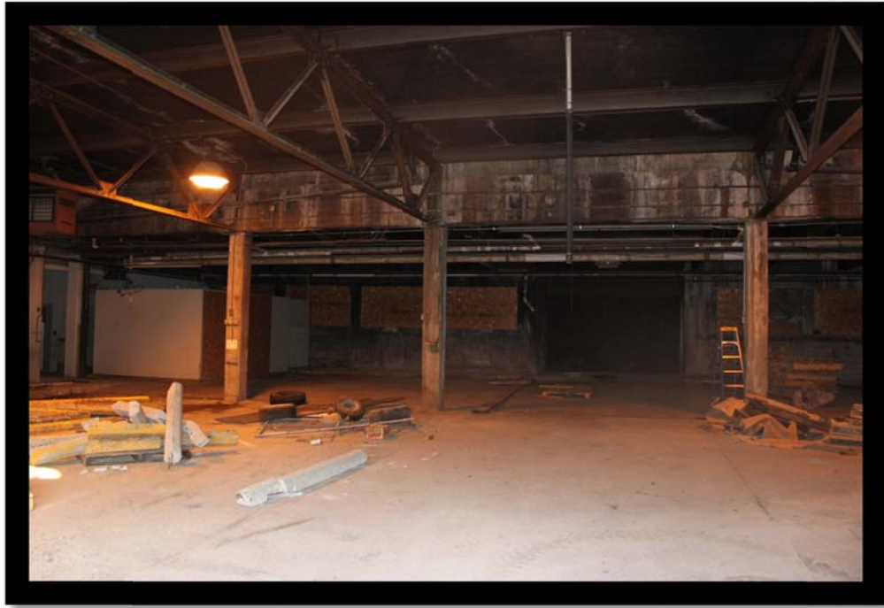
Looking north inside the North Garage
