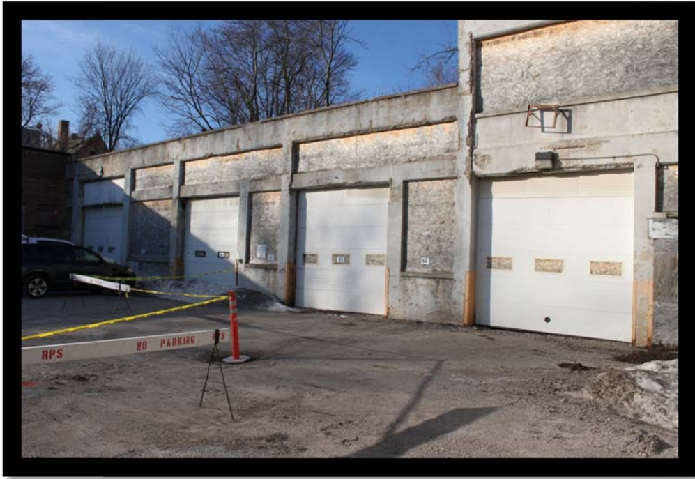
Looking southwest at the West Garage
