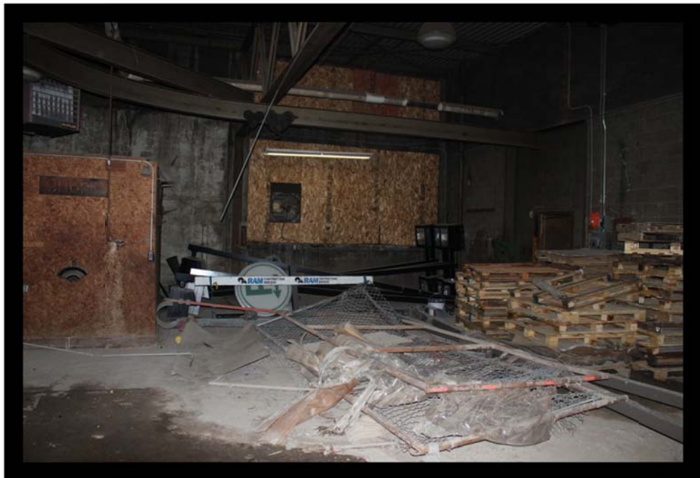
Looking west at the former carpentry shop inside the West Garage
