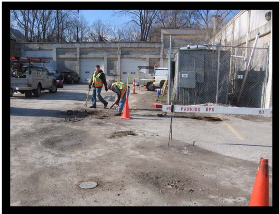
Looking west at West Garage, monitoring wells, piezometers, and manholes associated with the remediation system (right)
