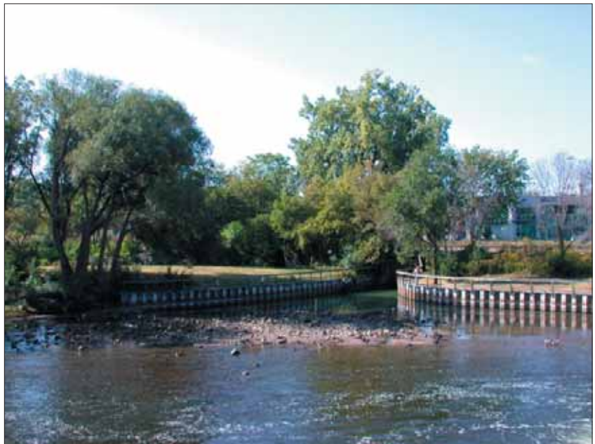
Allen Creek outlet to the Huron River
