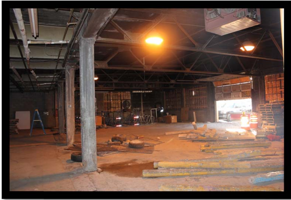
Looking east at the inside of the North Garage
