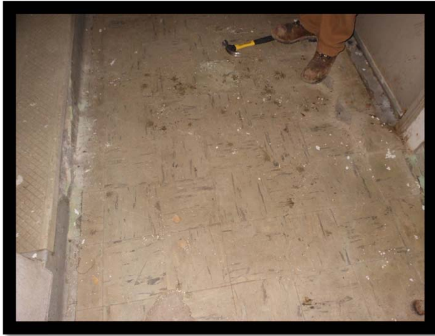
Potential asbestos containing tiles located in the offices above the North Garage
