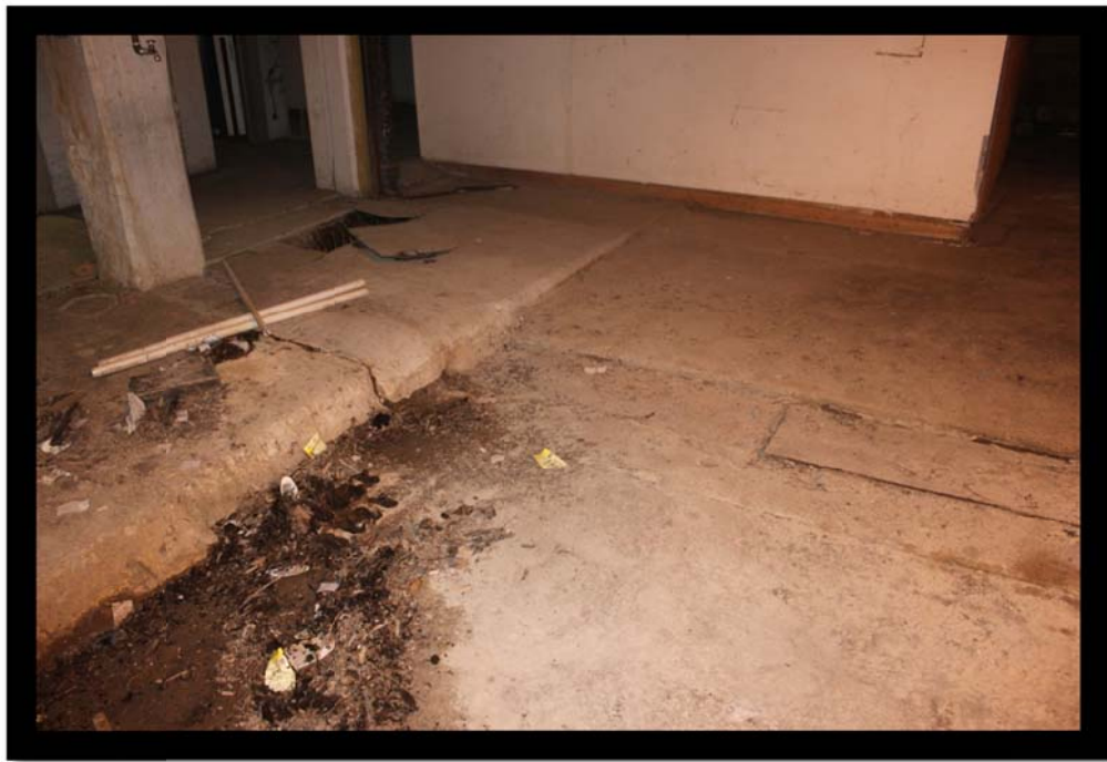
Trenches and drains located downstairs in the North Garage
