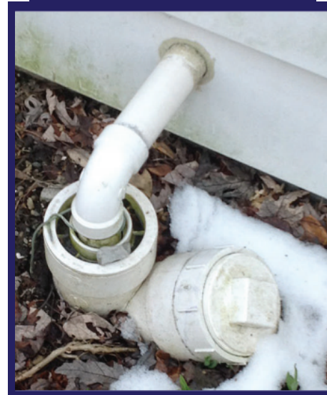
Pipe in Pipe Air Gap
