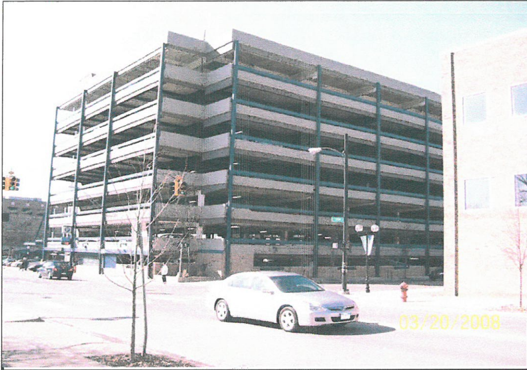
Figure 3.5 View of parking structure. Facing northwest.
