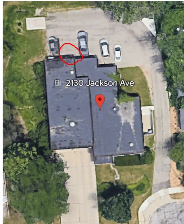
Ann Arbor Fire Station 3 (Ground Mounted Solar + Storage)
