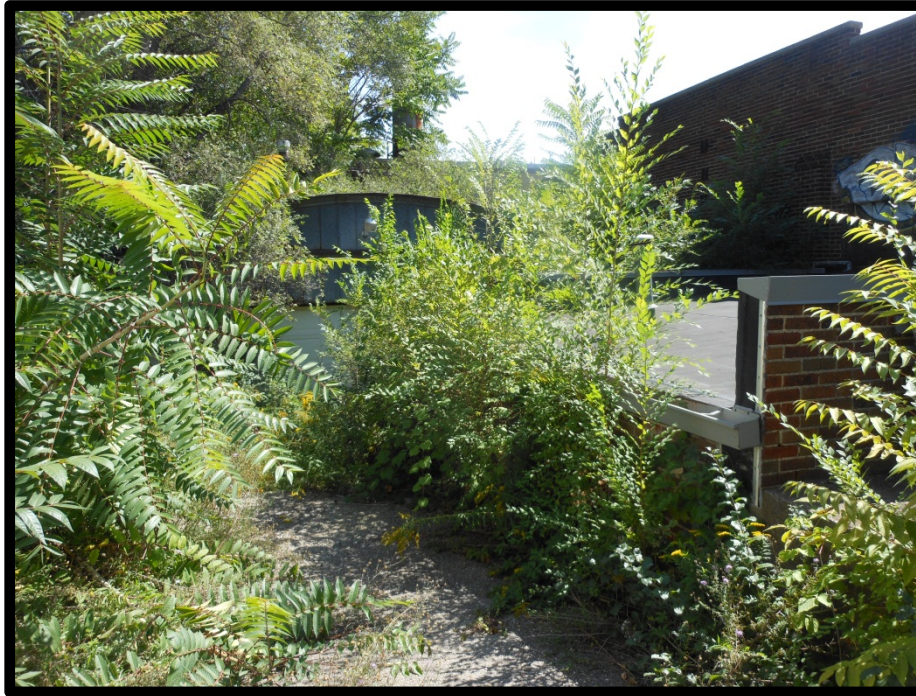
Looking east at the street maintenance garage (straight) and boiler/sump room (right).
