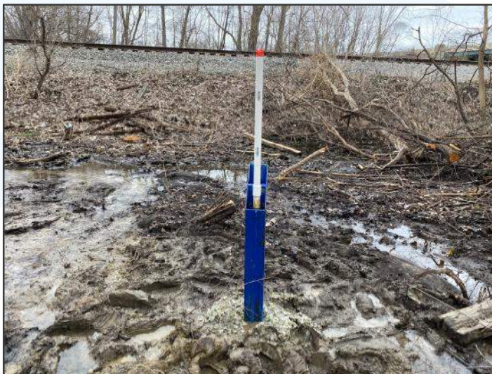
IMAGE 9: Photo of temporary observation well with additional casing. Photo taken April 1, 2022.
